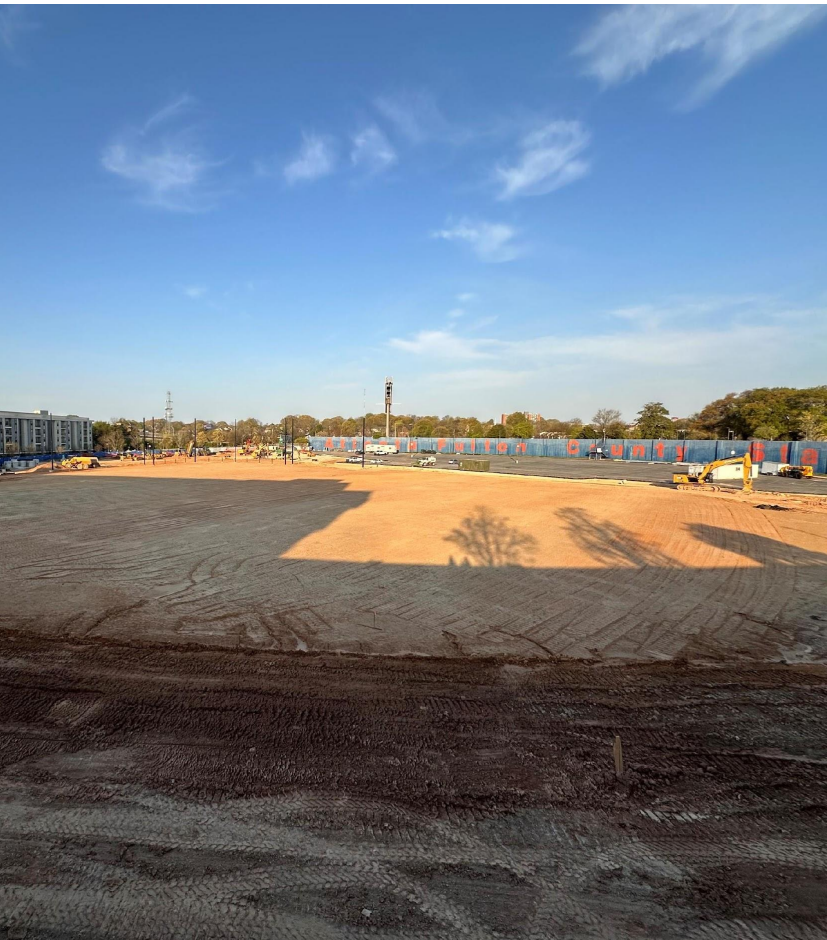
Pavement Stripped
