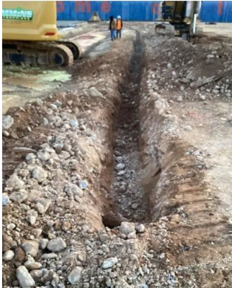
Rubble Debris in Fill
